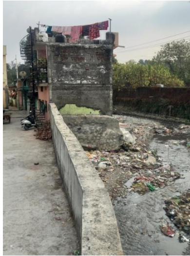
Fig. 6: Field photograph showing construction of building on the channel bed.
