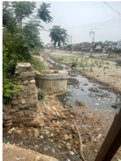
Fig. 7: Field photograph showing construction of sewage tank on the channel bed.
